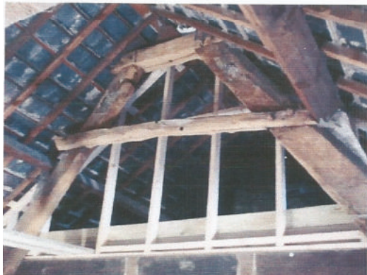
Cruck arrangement of roof beams
