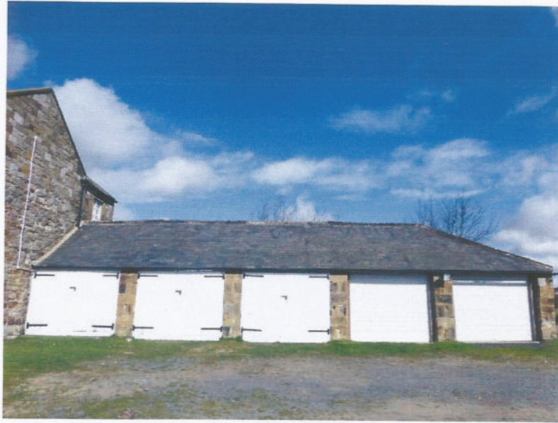
Cart shed attached on right, single storey, 5 bays with square piers and lintels
